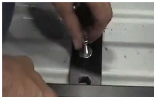
example of plusnut being compressed
